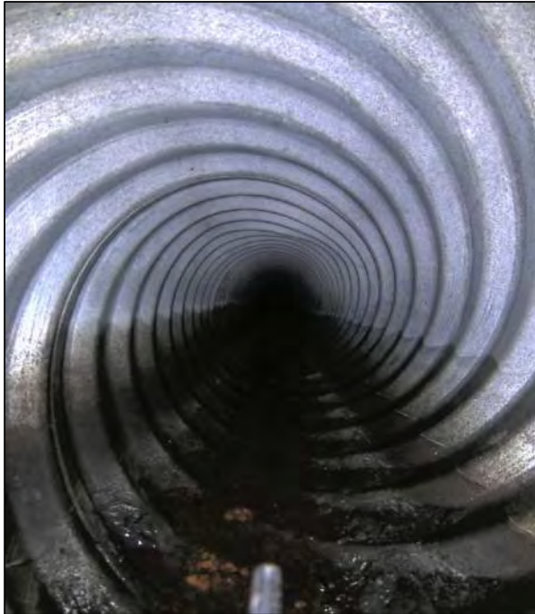
Image 1: Minor deformation at 1 o'clock position
