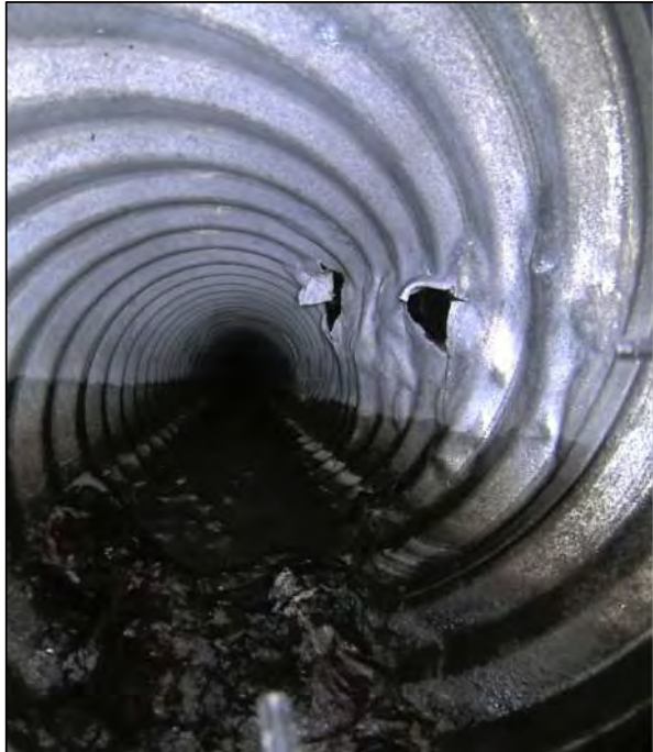
Image 2: Deformation and damaged pipe segment (holes) at 2 o'clock position
