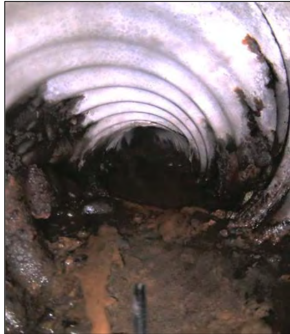
Image 2: Significant Grade Break
