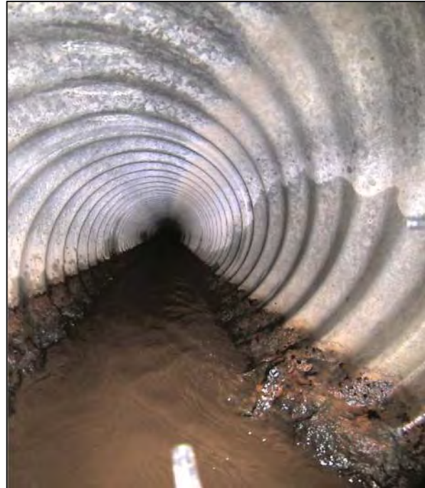
Image 2: Pinhole with Water Entering Pipe at 5 o'clock position
