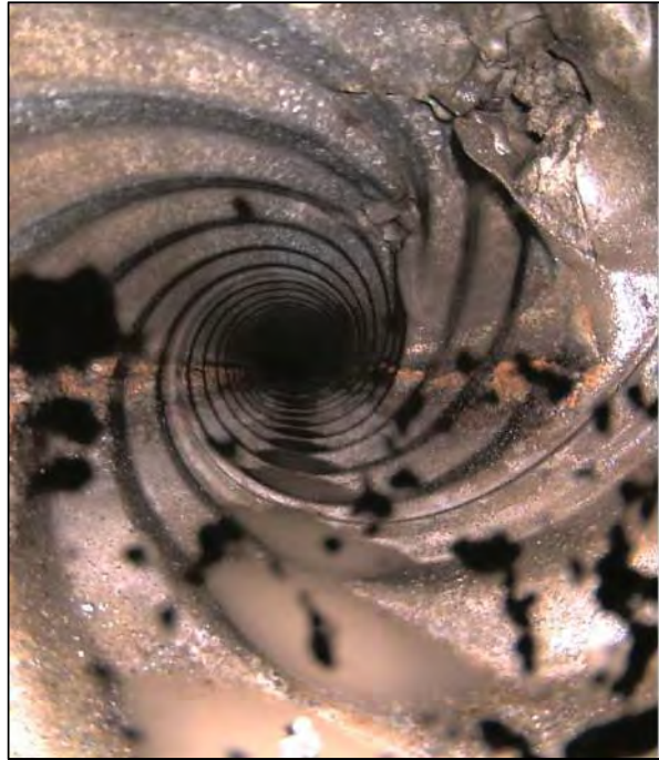
Image 2: Surrounding Soil & Rock Entering through Pipe Wall at 1 o'clock position
