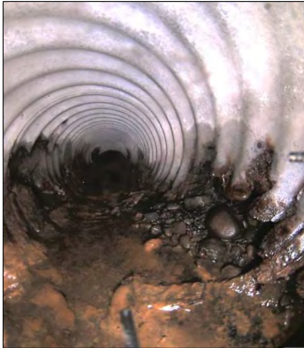
Image 1: Missing Invert and Pipe Wall, Surrounding Soil and Rock entering Pipe
