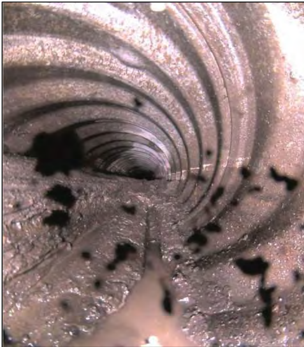
Image 1: Severe Debris present in Invert
