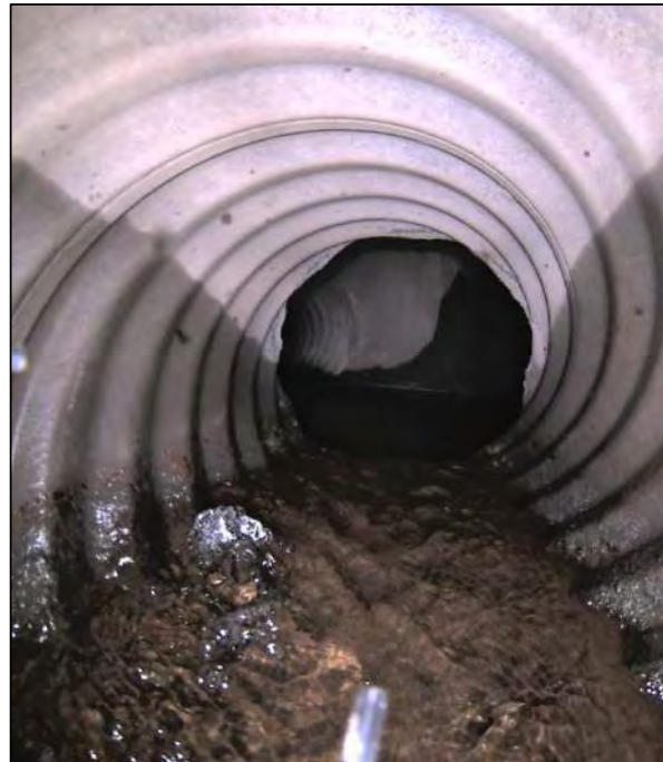
Image 2: Water entering pipe through hole at 8 o'clock position
