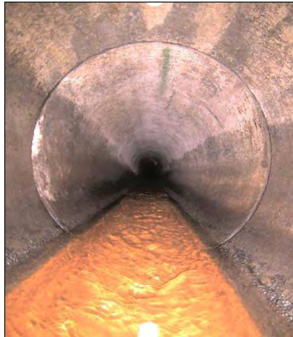
Image 2: Iron Deposits present in Pipe.
