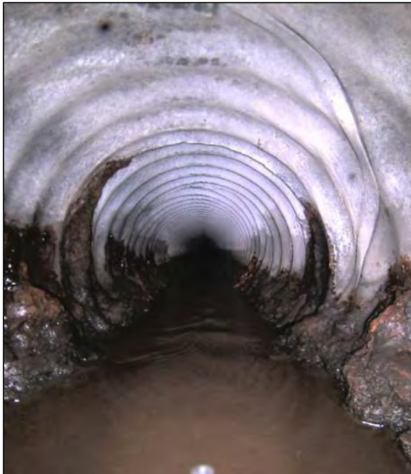
Image 1: Significant Infiltration and Buildup at Pipe Joints and along Walls
