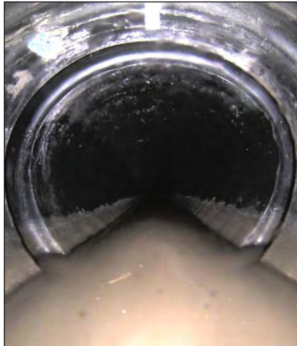
Image 2: Grade inconsistencies & Offset Joint
