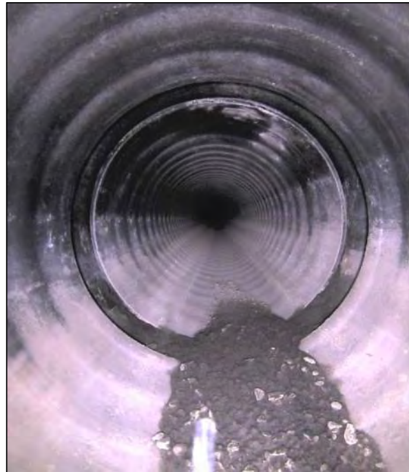
Image 2: Significant joint offset, no debris present upstream of joint
