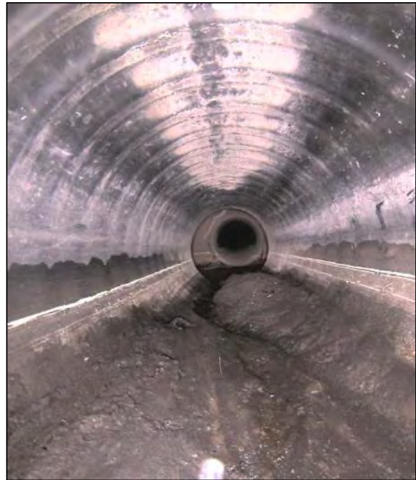
Image 2: Moderate debris buildup near manhole
