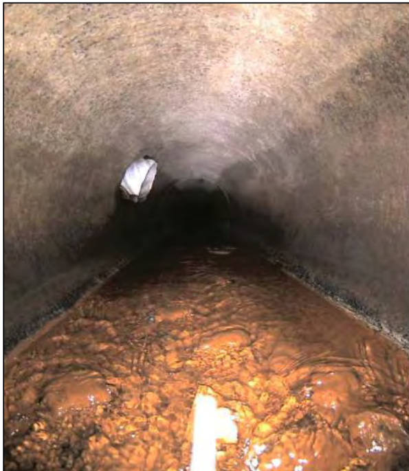
Image 1: Unmarked Lateral Pipe at 10 o'clock position
