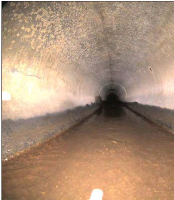
Image 1: Minor Longitudinal Cracks at 9 o'clock position
