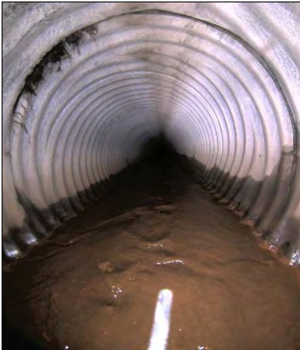
Image 1: Root Intrusion at 10 o'clock position
