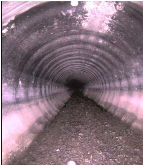
Image 1: Debris in invert, likely from joint offsets
