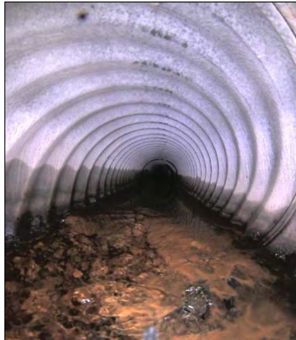
Image 2: Significant Debris in Invert
