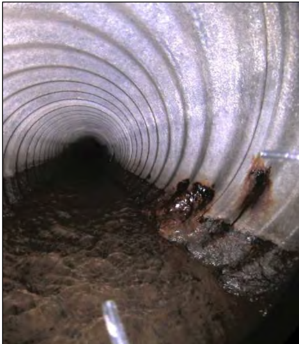
Image 1: Pinholes located at 4 o'clock position
