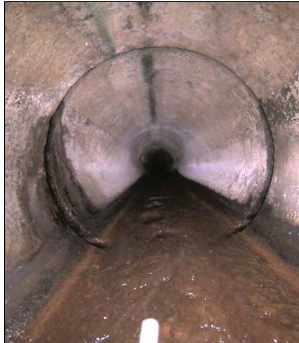
Image 2: Infiltration at Joint Offset
