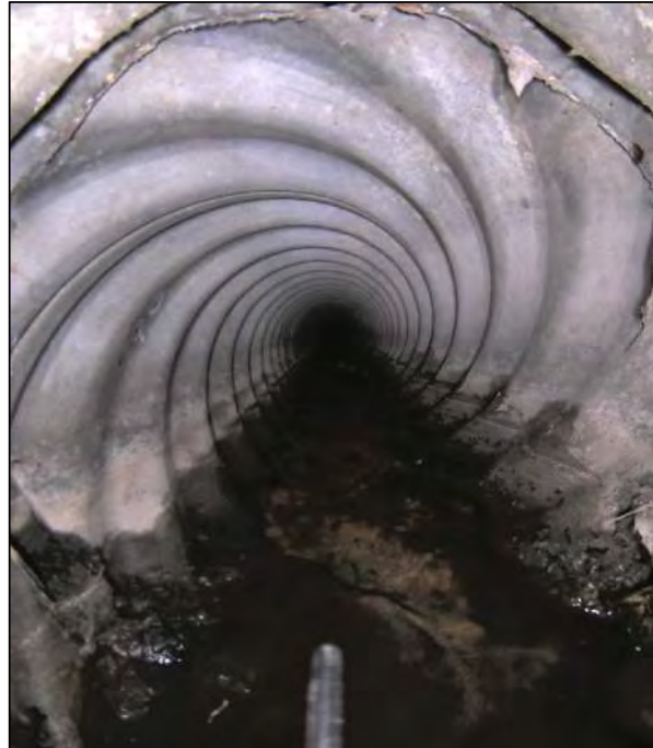
Image 2: Beginning of perforated section (on left side of image)
