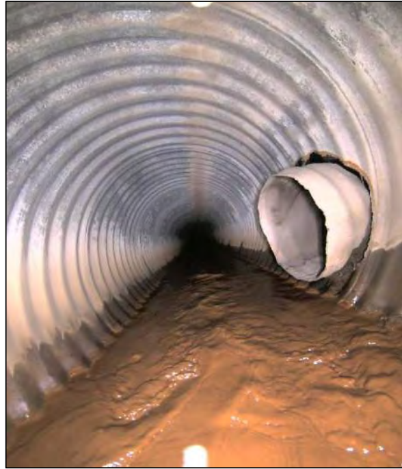
Image 2: Lateral Pipe at 3 o'clock position, significant debris/buildup in invert
