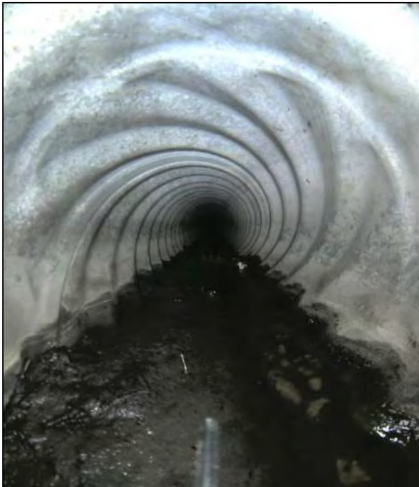
Image 1: Typical Pipe Condition, Debris present in invert
