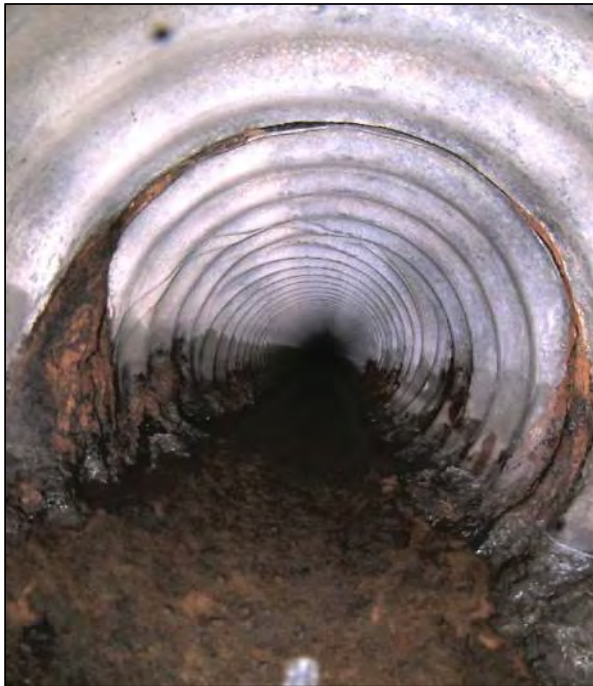
Image 1: Offset Joint & Infiltration
